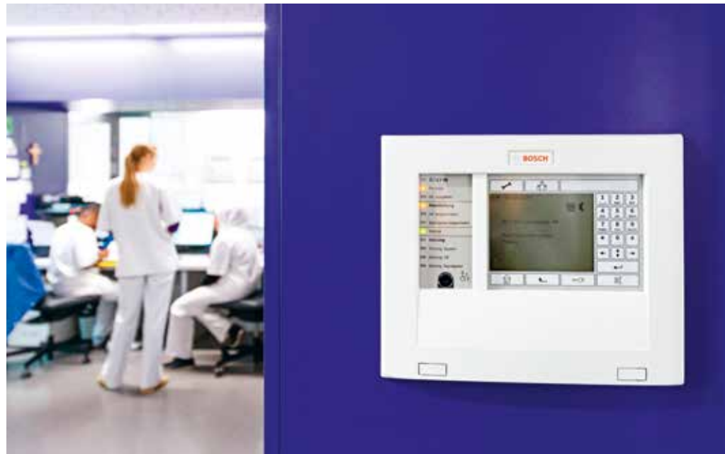
Each ward has a control unit for the fire alarm signals
